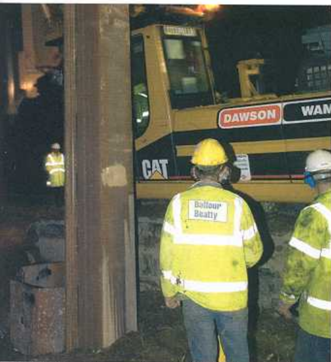
Sheet piles form a box section with high bearing capacity.
